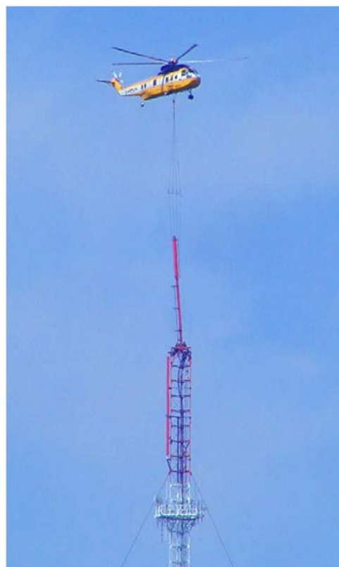
PSIMPTD-10-DCPA-46 BEING MOUNTED ON TOWER
