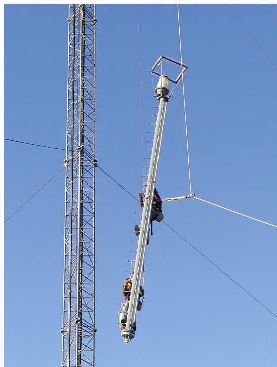
WDPB-DT ANTENNA BEING INSTALLED
