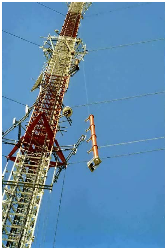
PSI ANTENNA BEING MOUNTED ON THE TOWER. PSI ANALOG CHANNEL 60 ANTENNA
